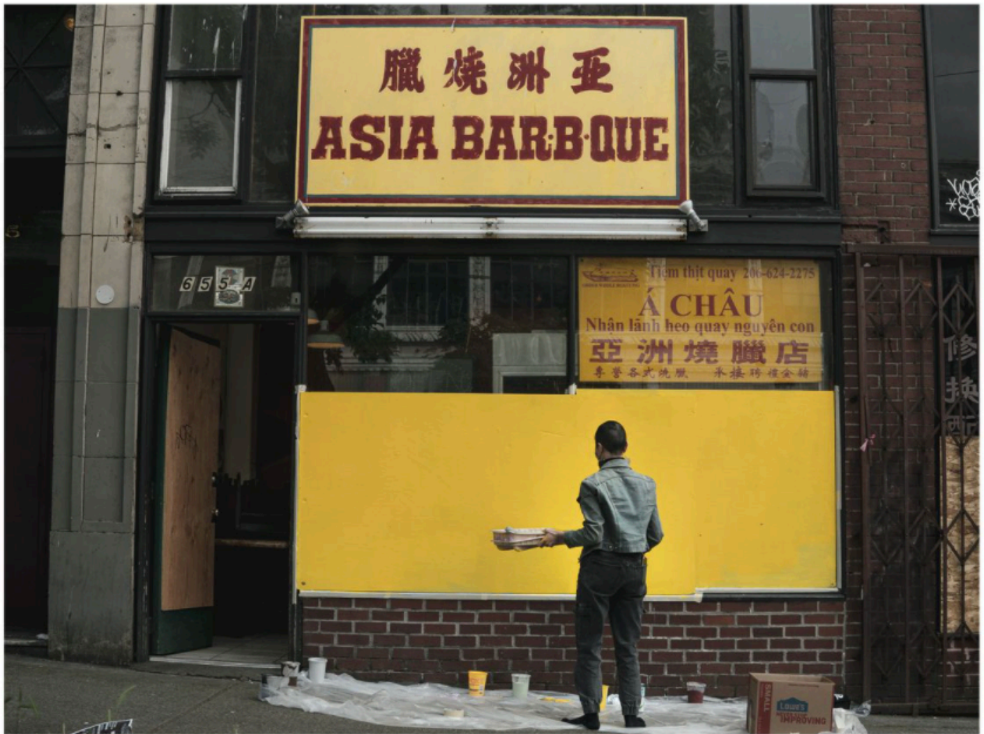
"Rebuilding" by Trevor Kwan
